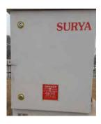
CCMS Panel provides the ability to the device to act as an interface between Street Light Controller (working over 2.4 GHz Mesh Network) and Surya IoT Platform.
